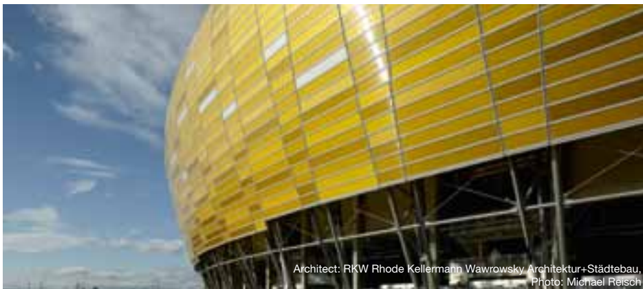
Figure 8: Examples of UV-protected, coextruded Makrolon® sheets
